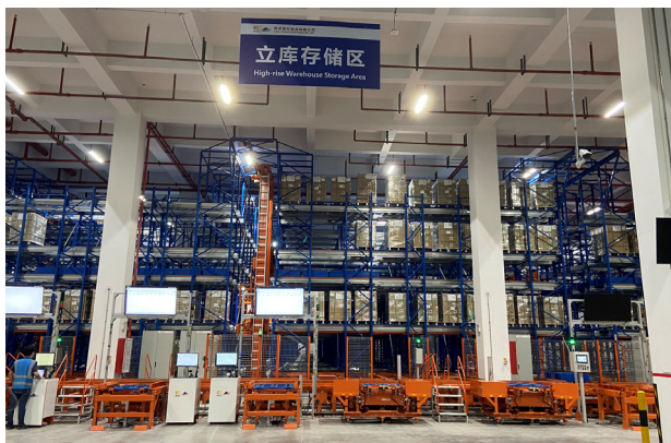
Densely tiered automated warehouse
